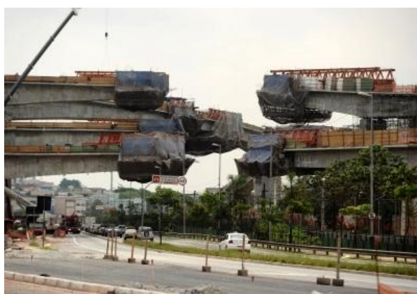
World Cup infrastructure works in Brazil PA.18498184
